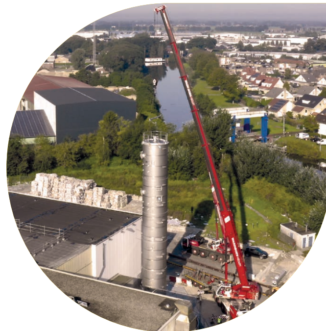
Installation of the Econvert plant for anaerobic wastewater treatment for biogas energy in Coevorden the Netherlands.
